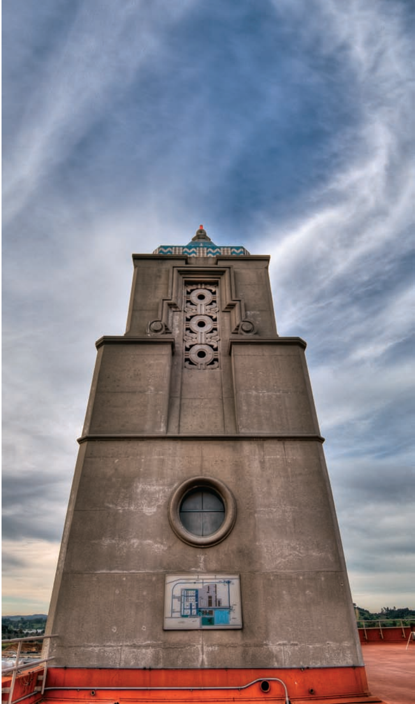
Metropolitan's F.E. Weymouth Water Treatment Plant in La Verne.
